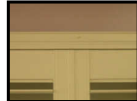
Double Check panels before securing.
