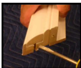
Insert screwdriver into slot under filler strip.
