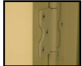
Hinge spacer installed
